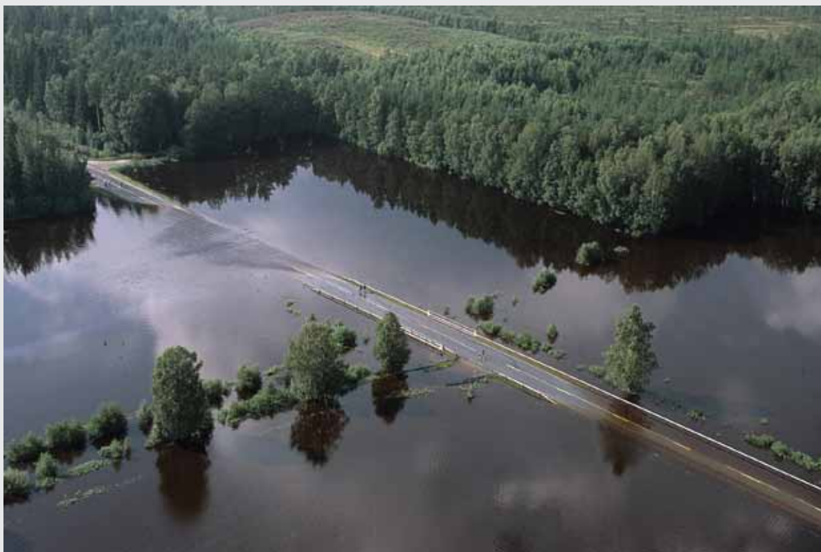
Photo: Flooding at Vöyrinjoki River (Finland) in summer 2004 © YHaphoto/Unto Tapio
