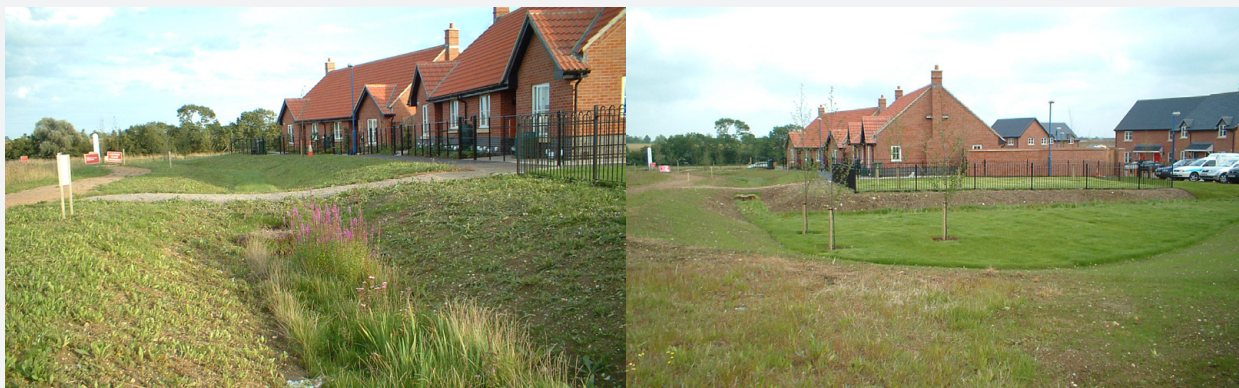
Photo 3.1 Sustainable urban drainage systems in Cambridge (United Kingdom)
