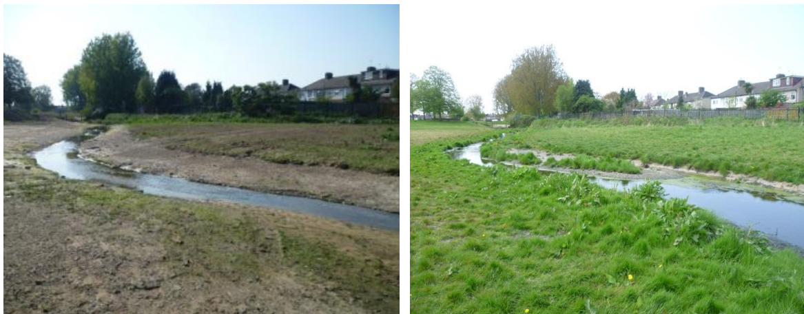
Picture 2: Reach 3 immediately after restoration in Autumn 2011 and Spring 2013. Two views show rapid morphological recovery from a newly restored channel to vegetated banks with mid channel bar formation. Source: Environment Agency.
