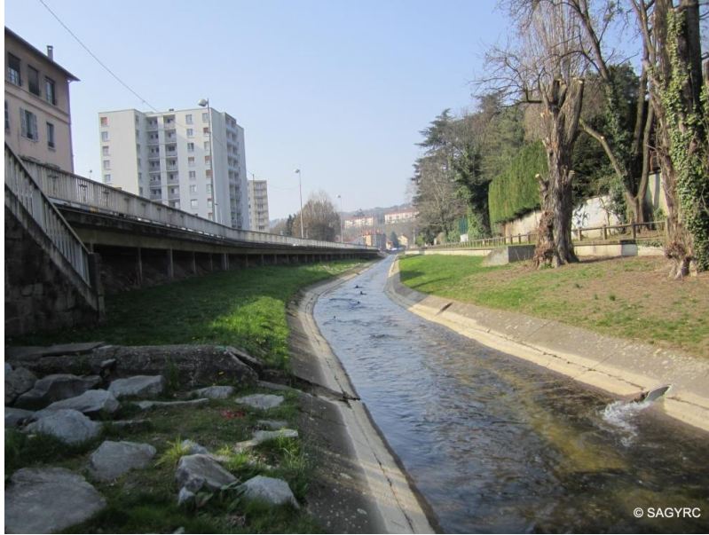
Site at Oullins before restoration in May 2014 (Source: SAGYRC).
