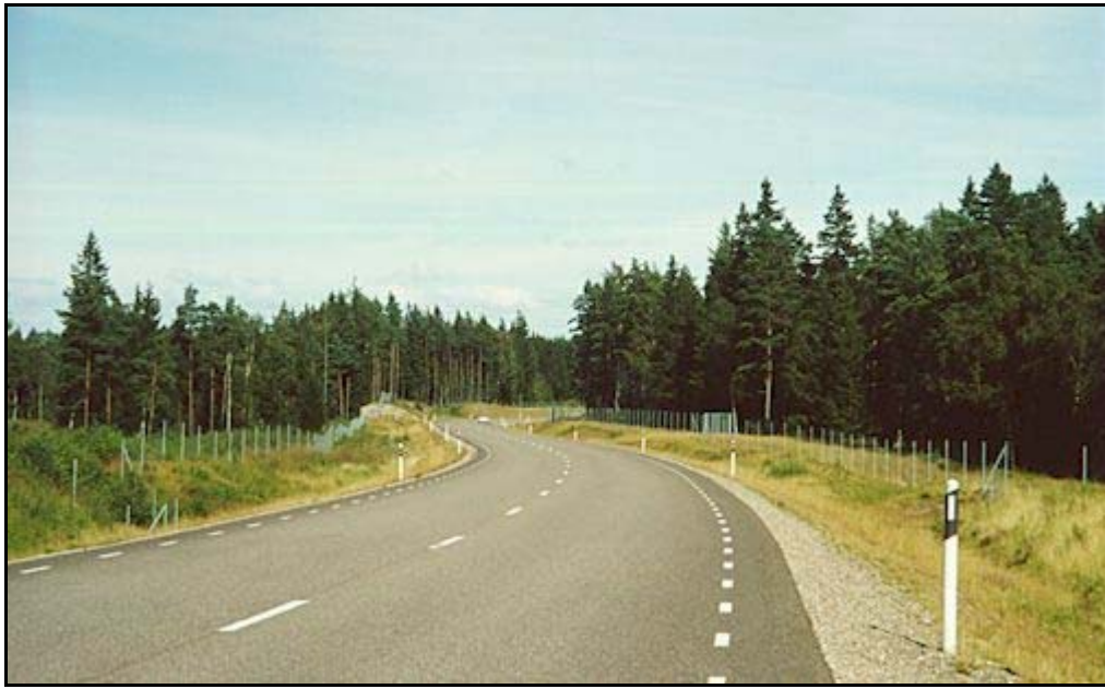
Photo: Road fencing in Sweden
