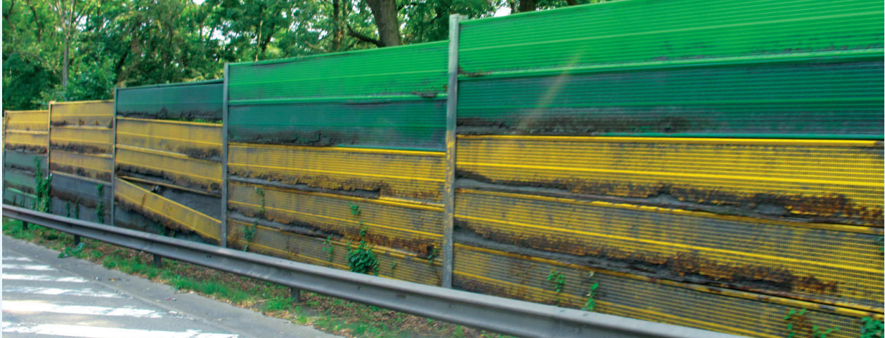
Image: © SPW Mobility and Infrastructures.
