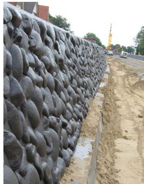
Fig 11: Low-level sound barriers
