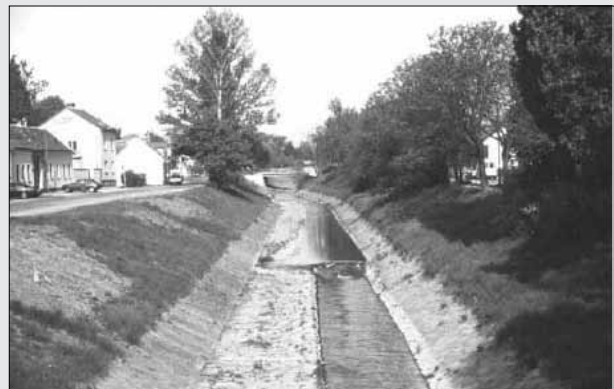
After the flood in 1954 the Liesing was pressed into a u-shaped concrete bed © Wiener Gewässer
