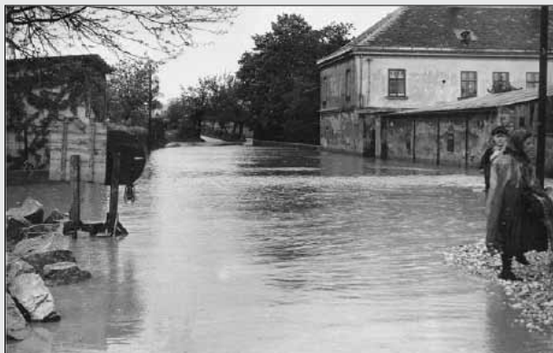
Heavy flood events in 1954 © Wiener Gewässer
